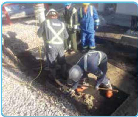
The contaminated Alabsorb layer was removed within the contamination area.
