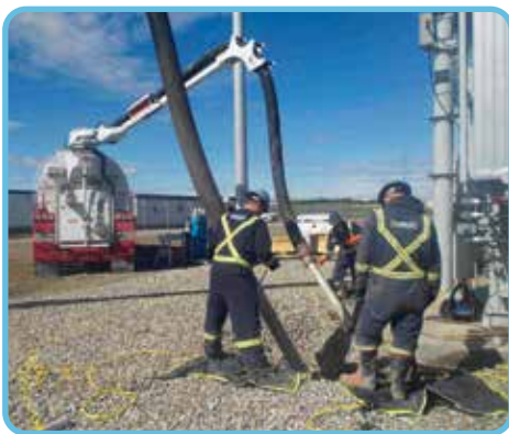
A Vac-Truck was used to remove all the contaminated stone.
