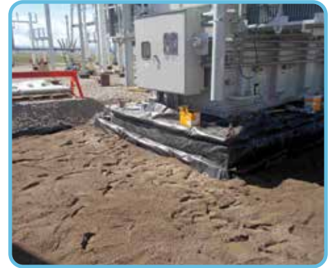
The remaining layers were re-installed.
