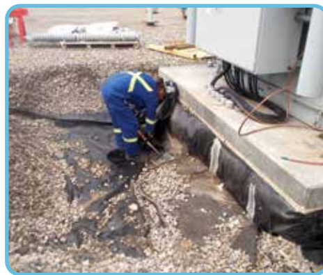
The impermeable liner within the contaminated area was inspected.
