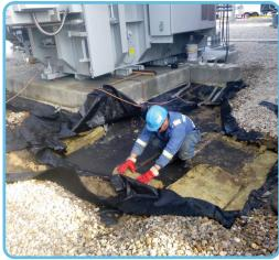
The nonwoven layer also showed signs of oil penetration in this area and was cut out (left), and turned over (right).
