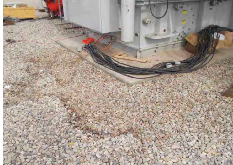
Visual discoloration was observed from the area that came into contact with the oil.
