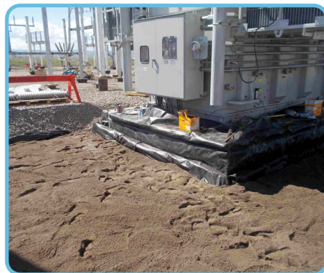
The remaining layers were re-installed.
