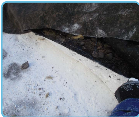
All the contaminated layers were removed until the clean Oilmats and Albasorb could be seen.
