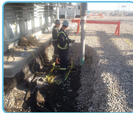
The existing non-woven geotextile showed signs of oil contamination, which was removed and discarded.
