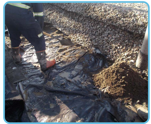
The top contaminated sand layer was removed within the contamination area using the Vac-truck.
