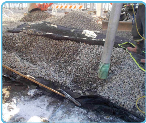
The construction crew removed and disposed of all the layers that came into contact with the oil.
