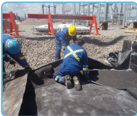
A new Oilmats was cut and placed, maintaining the required minimum overlap in between the existing and new Oilmats layers.
