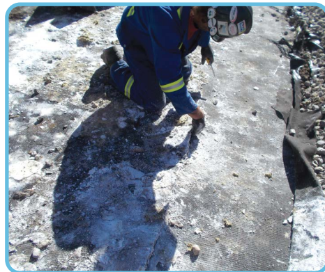
The contaminated Oilmats was removed and disposed of by the construction crew.
