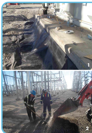
1. The sand beneath the congealed oilmat was observed to be clean and unaffected by the spill. 2. Stone was replaced in the affected area. 3. The site was cleared of all debris and all equipment was removed from the substation.
